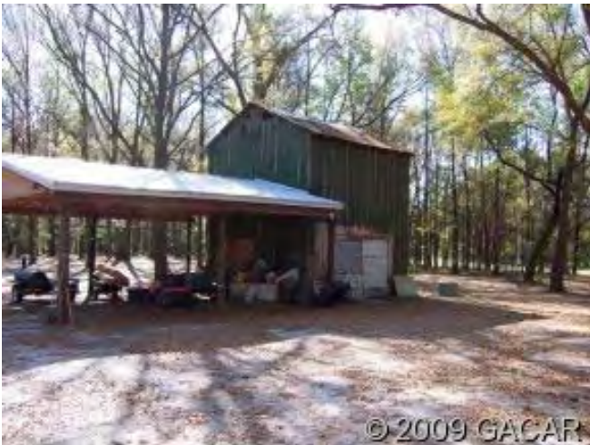
Pole barn and storage
